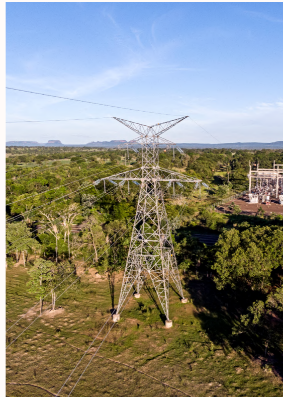
BTE Transmission line
