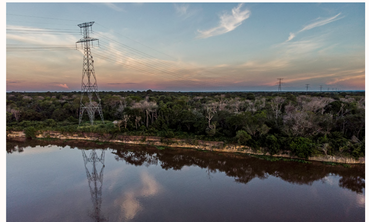
Corumbá transmission line
