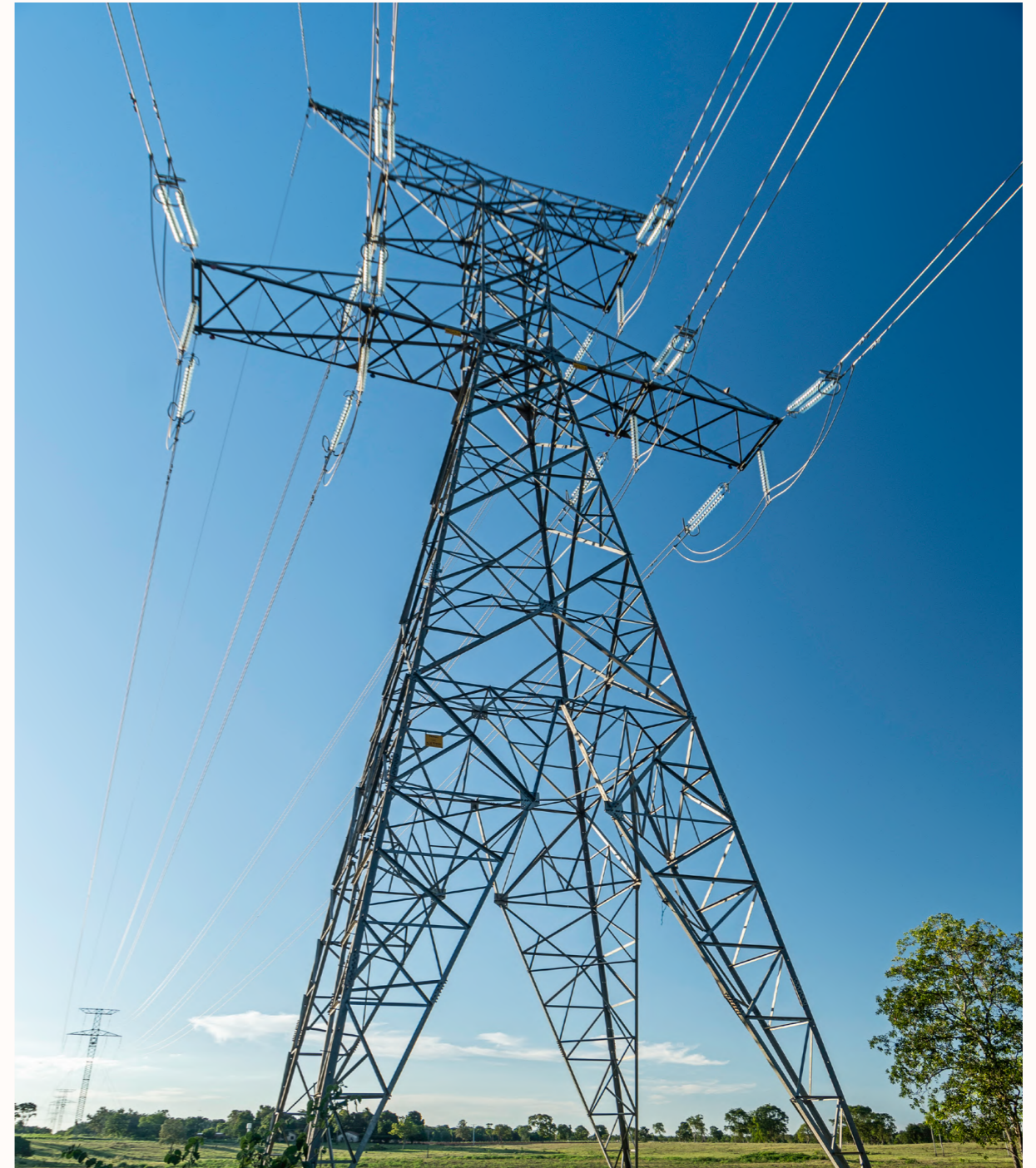
Jaurú transmission line
