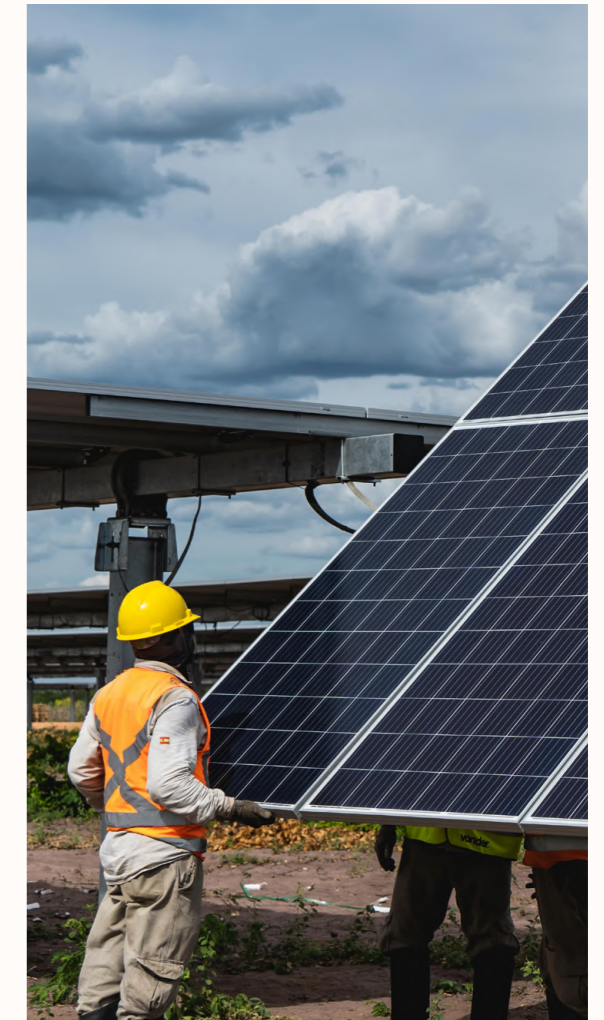
Maintenance work in UFV-SJP
