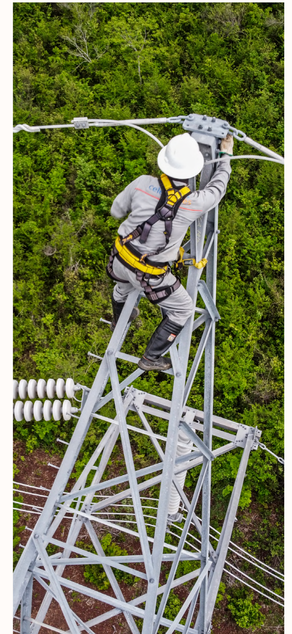
Maintenance work in SITE
