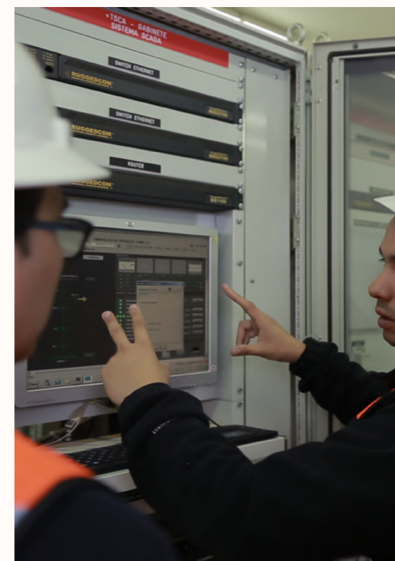
Maintenance work in Hualqui substation
