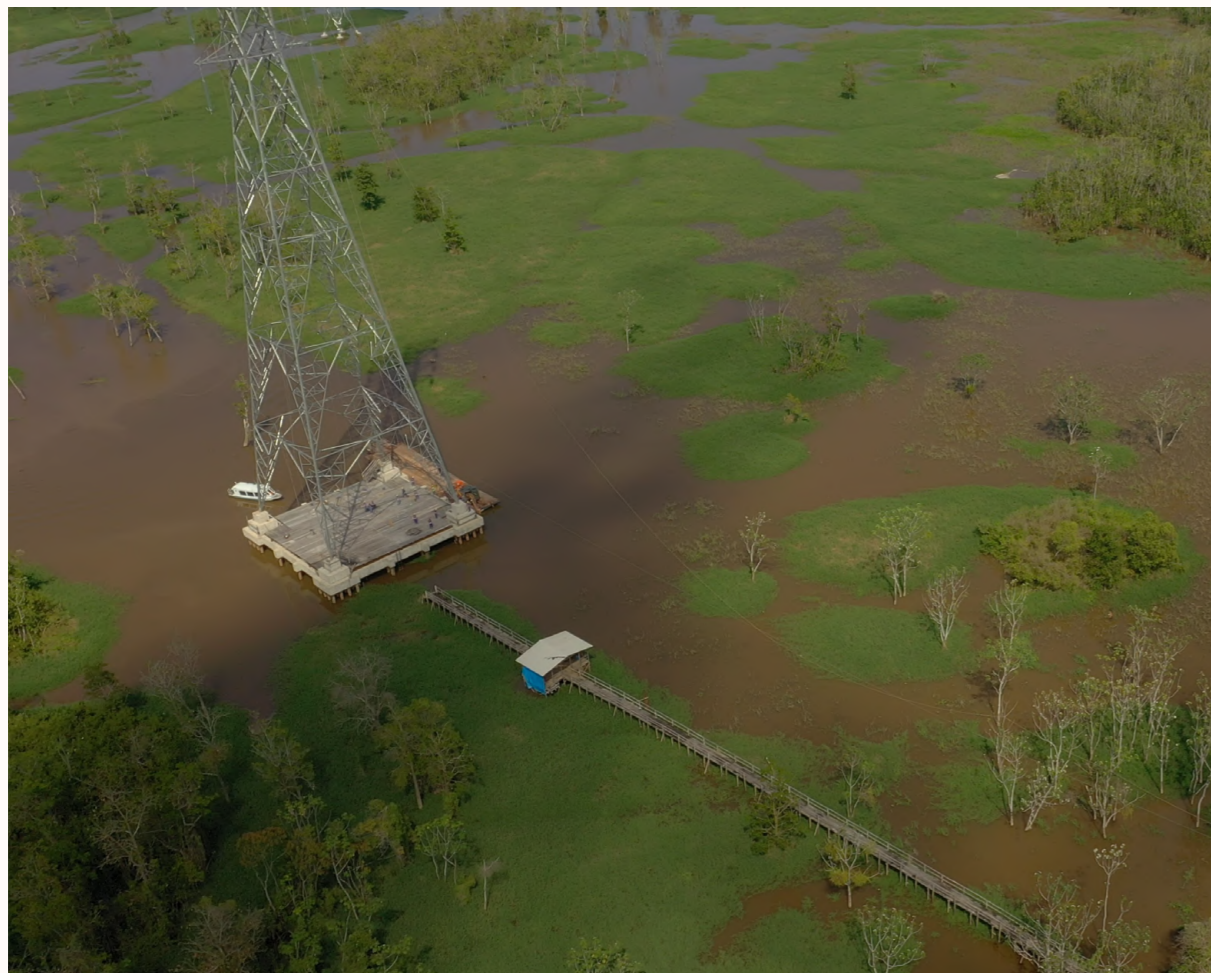
PATE Transmission line
